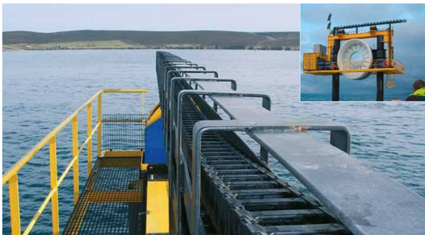
The maintenance-free series 4040HD protects the igus® chainflex® motor and signal cables during the lifting and lowering movements of this tidal turbine and protects them against the aggressive ambient conditions. 20m vertical movement above and below water
